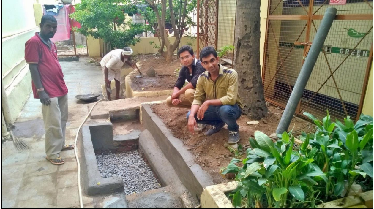
Consruction of Rain harvest pit: 6/7/14 to 8/7/14
